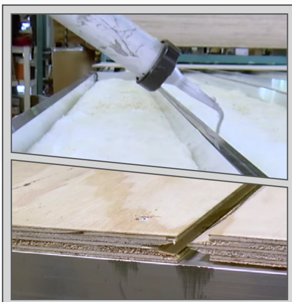
GLUED & SCREWED PLYWOOD FLOORING 5/8" Tongue & Groove Plywood Floors Glued & Screwed on Aluminum Floor Joists (16" on Center)
